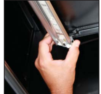
2. Pinching the latching clips inward at the ends of the luminaire, rotate luminaire up at each end until hooks are free, then remove.
